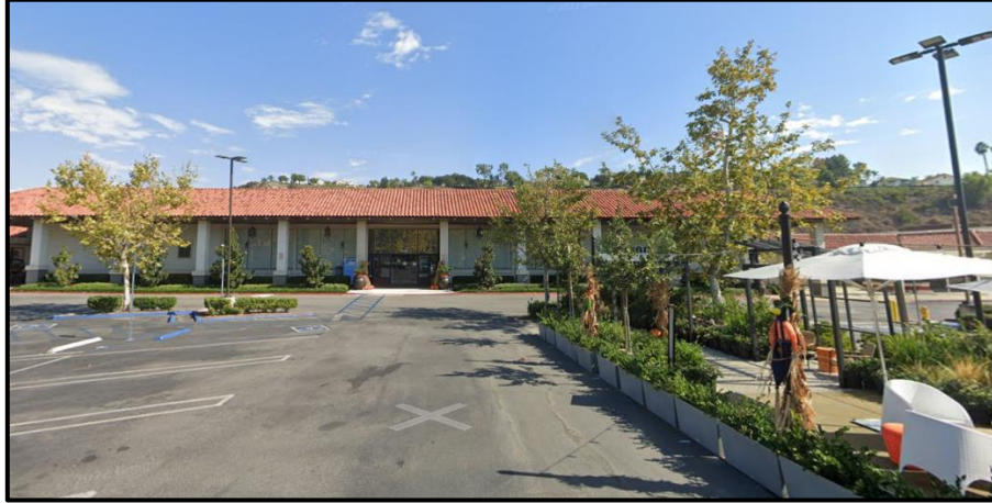
View looking east towards MART and North Paseo
